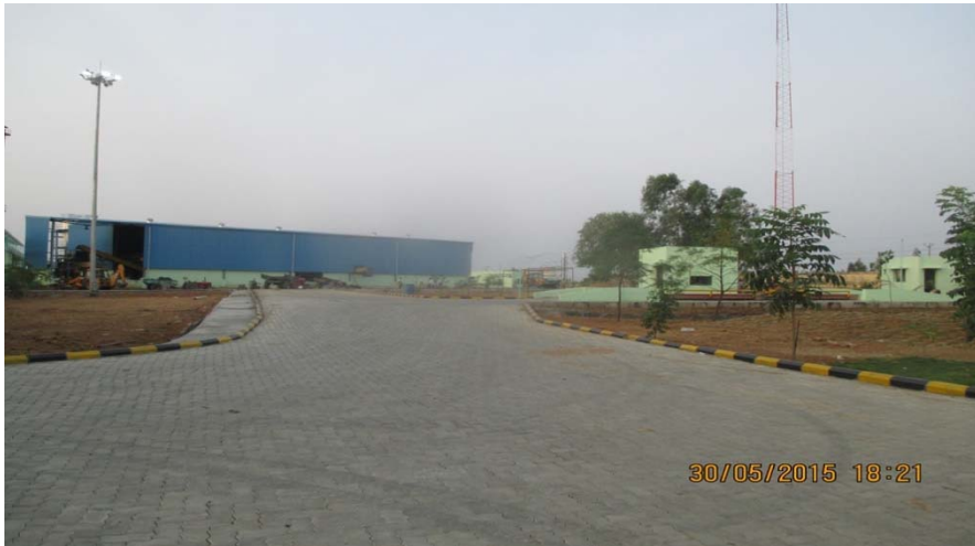
OVER ALL VIEW OF THE PLANT
