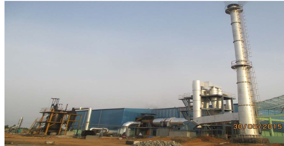
DRYER AND HOT AIR GENERATOR
