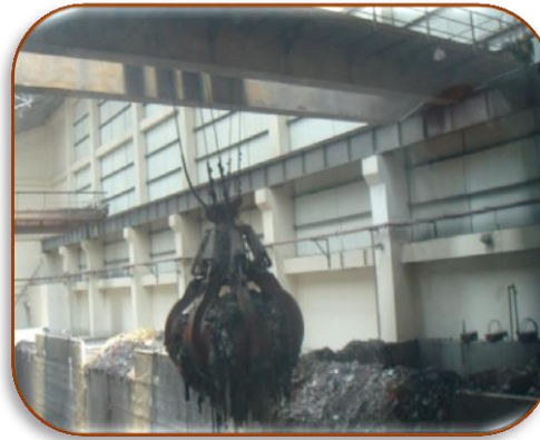
Lifting with Grab Crane
